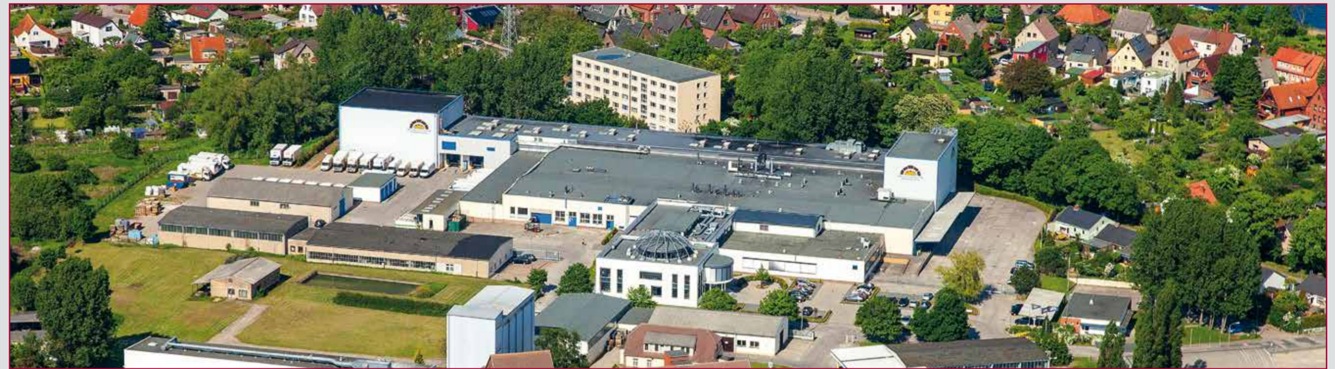
View of entire bakery facility
