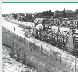
Construction of the railway route and the Schwerin causeway, 1975
